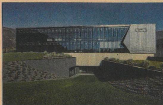
Factory and Headquarters, Pove del Grappa (Venezia)
